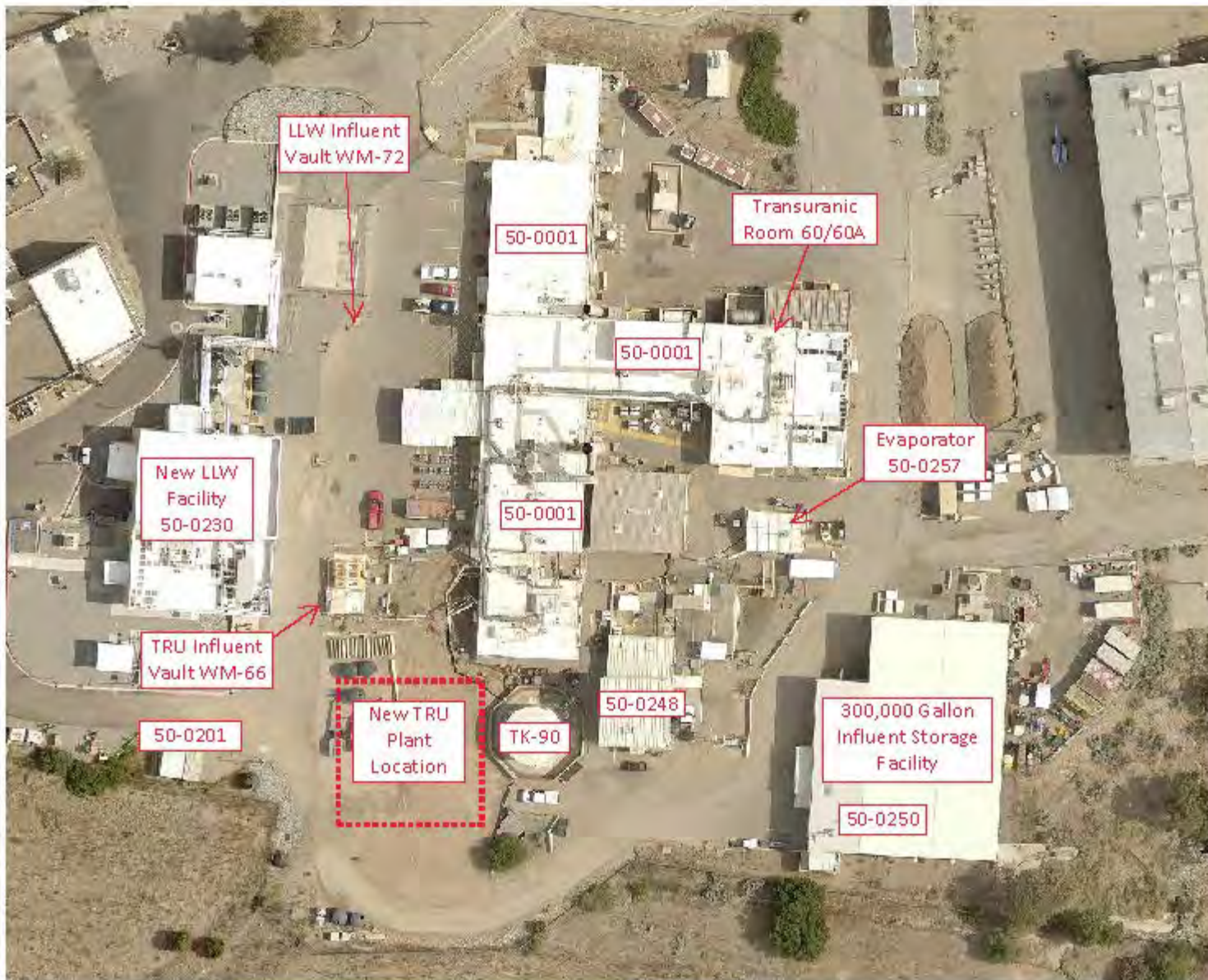
Figure 1. Aerial View RLWTF
